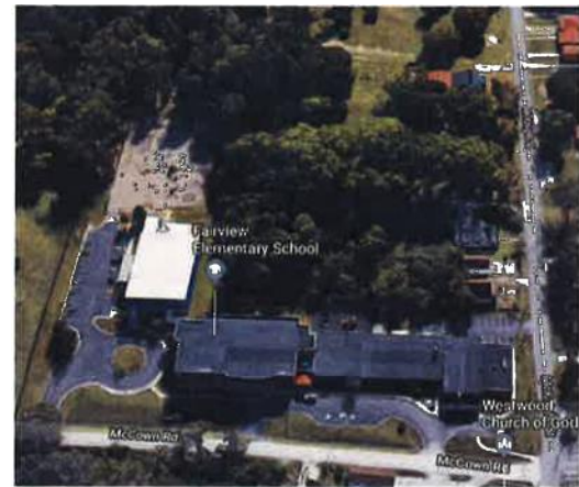
Lawn Care Service-Fairview Elementary School
